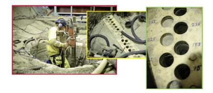
Fig. 2-12 Core drilling of the buffer. A template was used to obtain the correct position of the cores (SKB, 2012)
