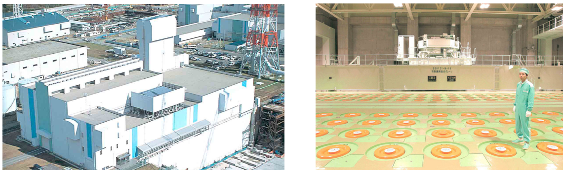
Figure 1-2(a): JNFL Vitrified Waste Storage Center (left) and HLW storage pits (right) (photos: courtesy of JNFL).
