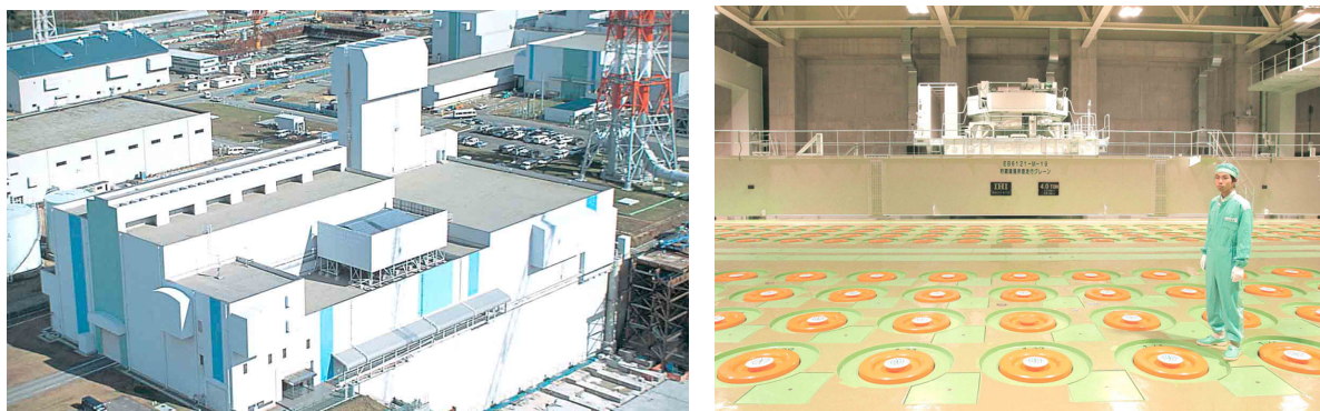
Figure 1-2(a): JNFL Vitrified Waste Storage Center (left) and HLW storage pits (right) (photos: courtesy of JNFL).
